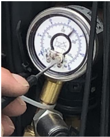
Figure 6 Adjusting of condensing pressure on the left. On the right graph and table decreasing condensing pressure at the approximately same outside temperature 25,5+0,5°C also evaporating pressure, temperature and cooling performance have decreased and EER has increased
